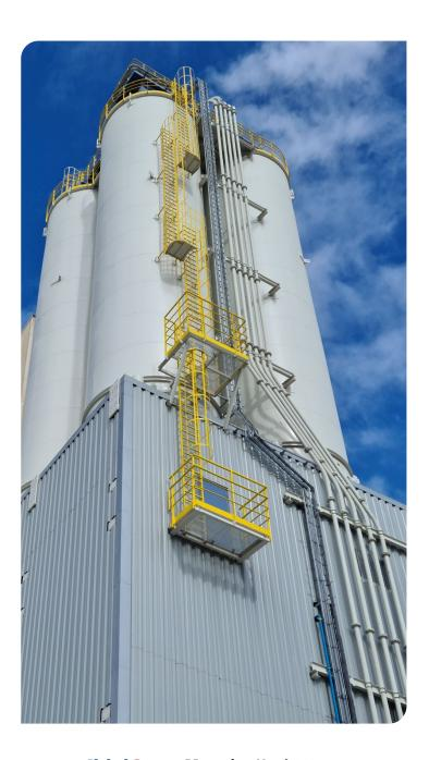
Biko-Serwis was asked to design and build an HRB blending plant by Carmeuse for a site in Belgium. The installation's main product was to be HRBs produced according to EN 13282-1 and EN 13282-2 standards, as well as composite cements according to EN 197-1 and limes according to EN 459-1. Depending on the selected recipe, the finished product may consist of: lime, cement, slag, fly ash and gypsum, as well as other additives. The assumptions and requirements specified were:
